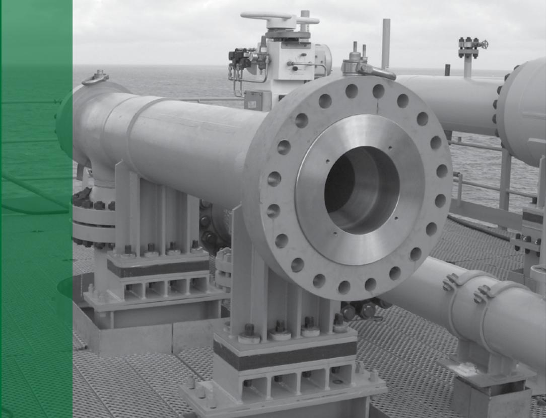
“ the gas ejector gave us about a 15% increase in production and we didn't need to install the extra compressor.
