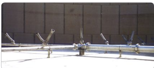
Multiple Jet Mixers installed on a manifold
