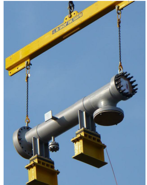
Transvac Ejector being installed onto Rig
